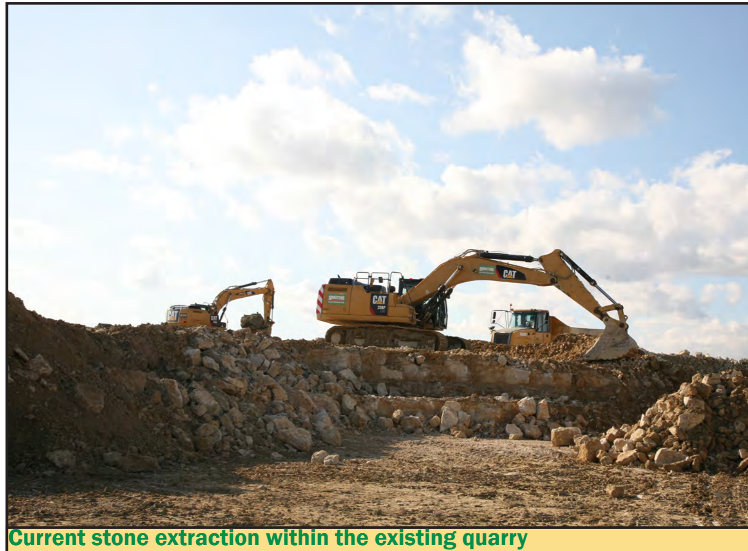
Current stone extraction within the existing quarry
